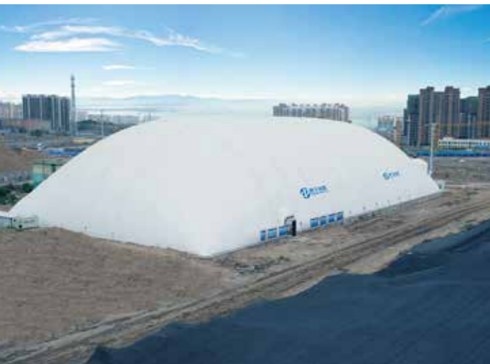
Project Site of the Xinjiang Zhongtai Chemical Soil Remediation Project
