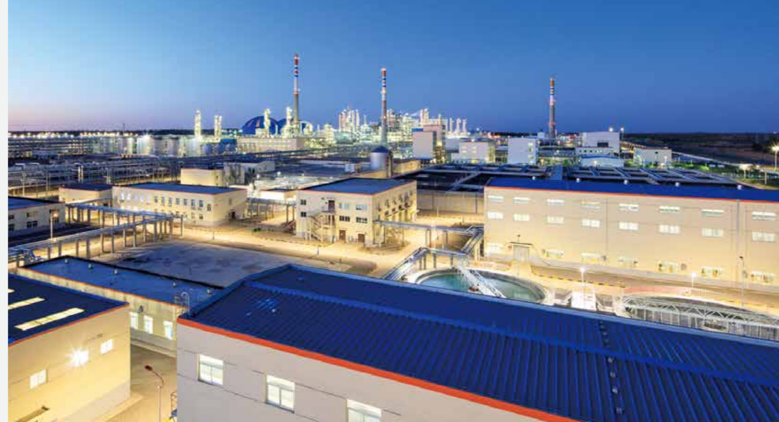
Wastewater treatment facilities for the Yankuang Yulin million-ton indirect coal liquefaction demonstration project, Shaanxi Future Energy Chemical Industries Co., Ltd.
