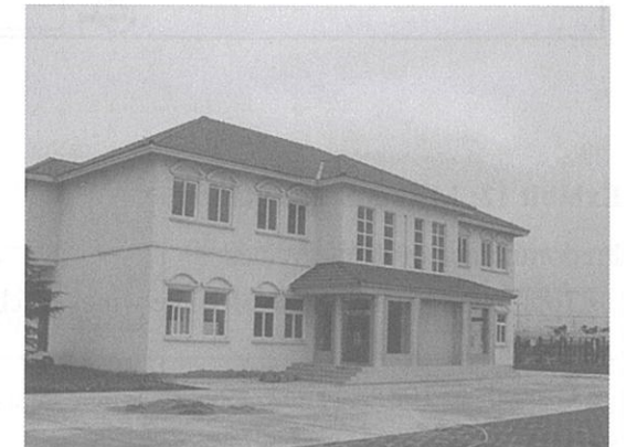
Exhibit 9: View of the New Office Building
